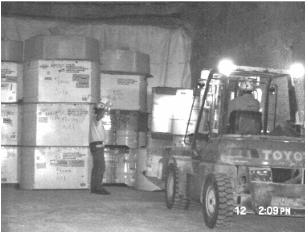
Figure 3. Waste being emplaced in Panel 1. Note stacks of three containers with MgO on top of each stack.
